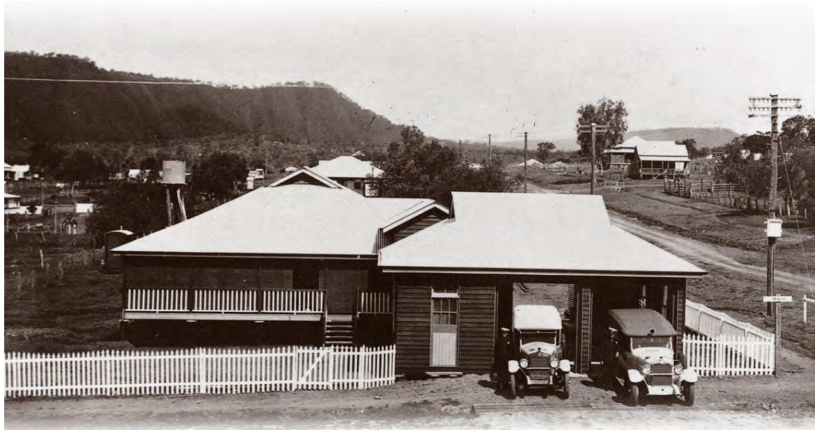
Centre building opened 1927
