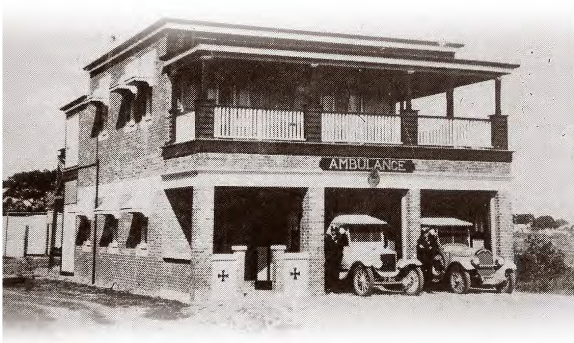
Townsville Rd Centre erected in 1927
