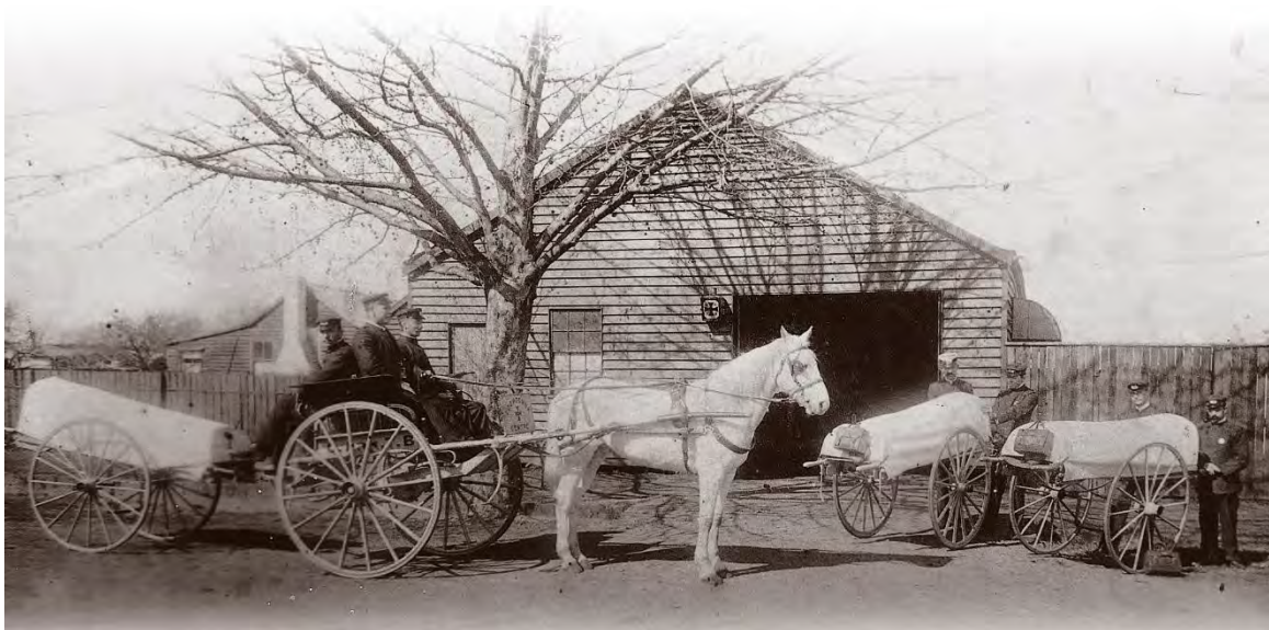
First ambulance building
